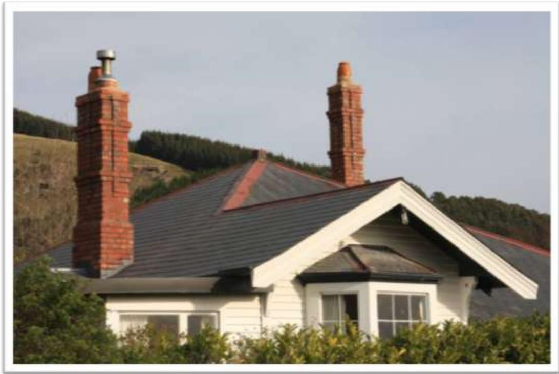
**Fig. 4:** Examples of brick veneer Quake Safe chimney's fitted in Canterbury
