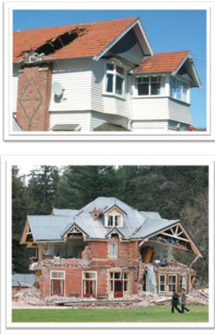
**Fig 2:** Extreme damage caused by Canterbury Earthquake 2010
